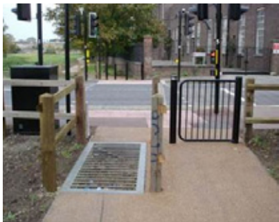
Animal grid and accessible gate incorporated in segregated entrance to shared cycle route and footpath
